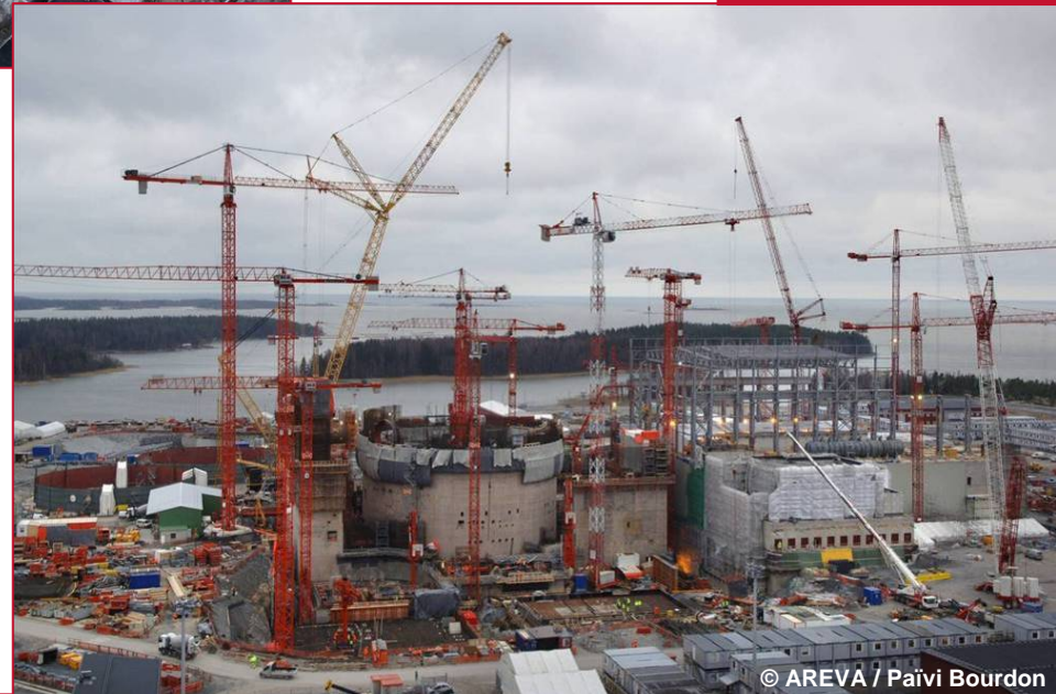
OL3 construction site
