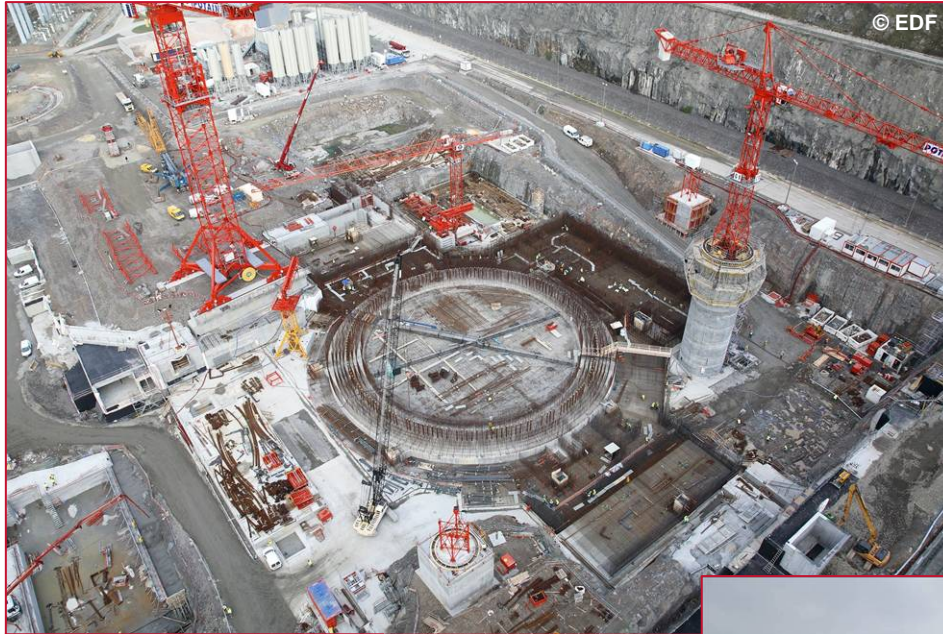
FA3 construction site
