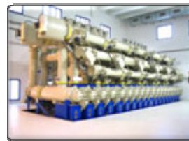
Gas-insulated substation
