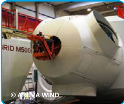
Assembling wind turbine nacelle
