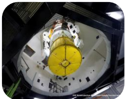
Flammanville 3 EPR (France)
