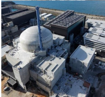
Chantier Flamanville 3 (France)
