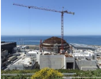
Chantier Flamanville 3 (France)
