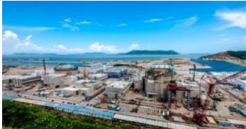
Chantier Taishan 1&2 (Chine)
