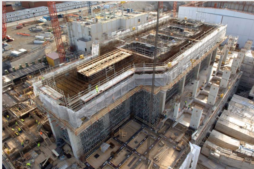
Turbine building next to the reactor building
