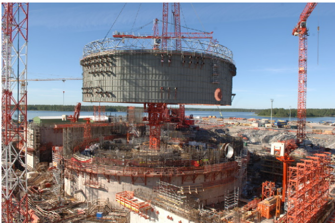
EPR construction site (TVO), June 2007, Olkiluoto, Finland
