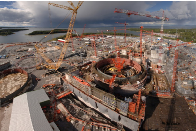
EPR construction site (TVO), September 2007, Olkiluoto, Finland
