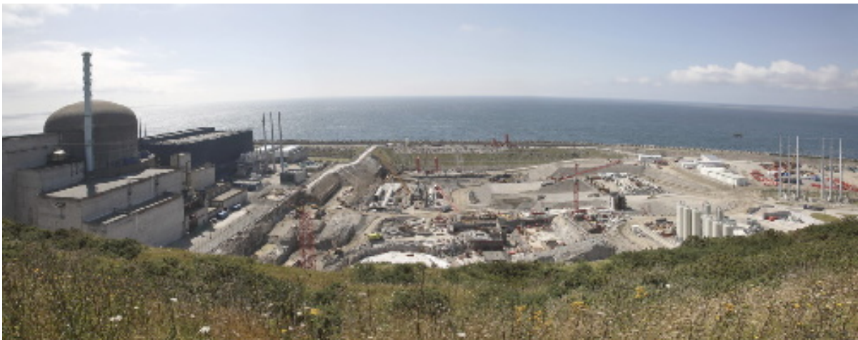
EPR construction site (EDF), July 2007, Flamanville, France
