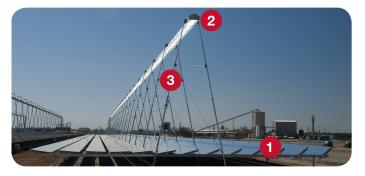
1/ Flat mirrors reflect sunlight onto a linear receiver above the mirror field.
