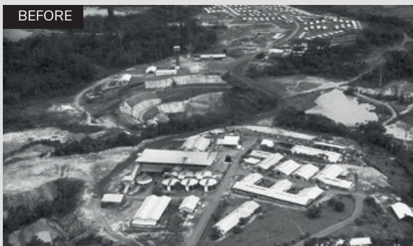
Processing plant at the Mounana mining site, Gabon
