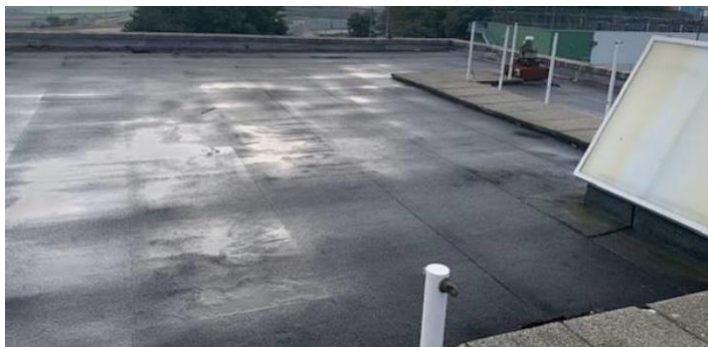
Roof of the utility building, East view
