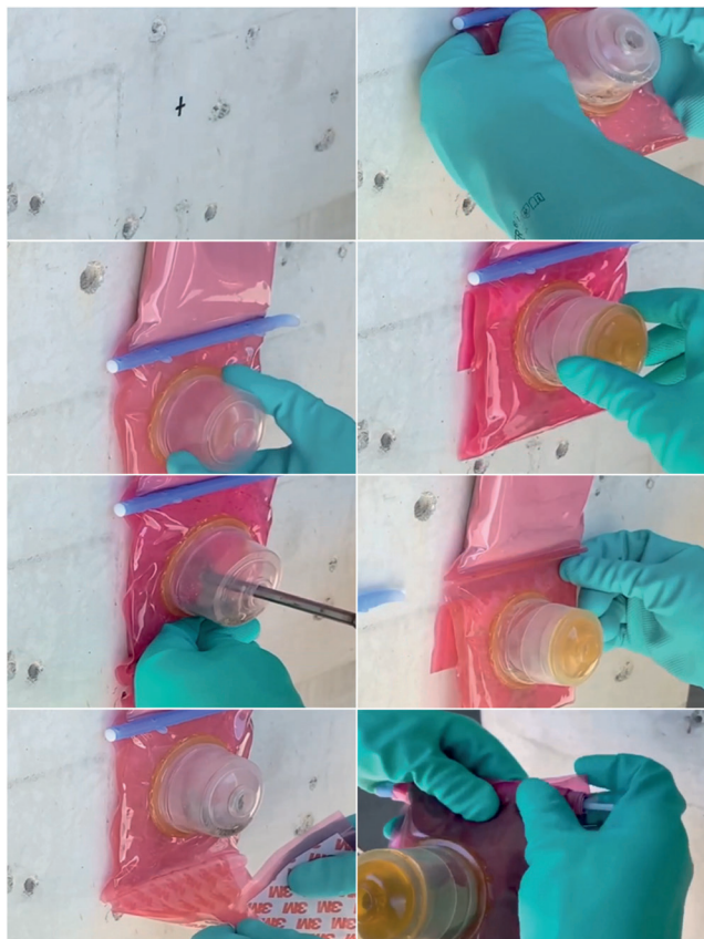
Drilling sequence with the EGPN solution
