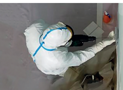
Drilling with the EGPN solution
