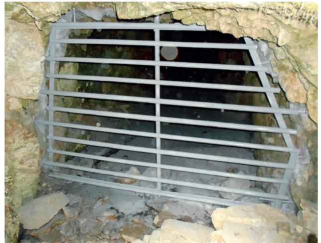
The grille is used to secure the entrance to a former mining gallery, sized to allow the bats to pass through
