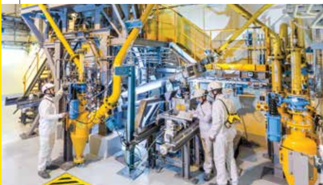
Conversion services carried out at our facilities in France for our customers worldwide.
