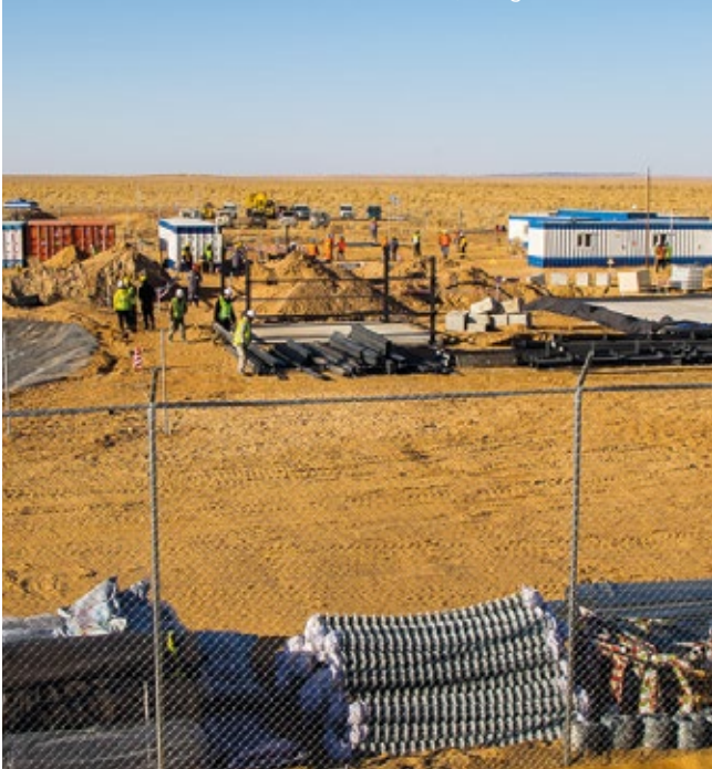
Zuuvch Ovoo ISR Pilot's construction works, Mongolia.
