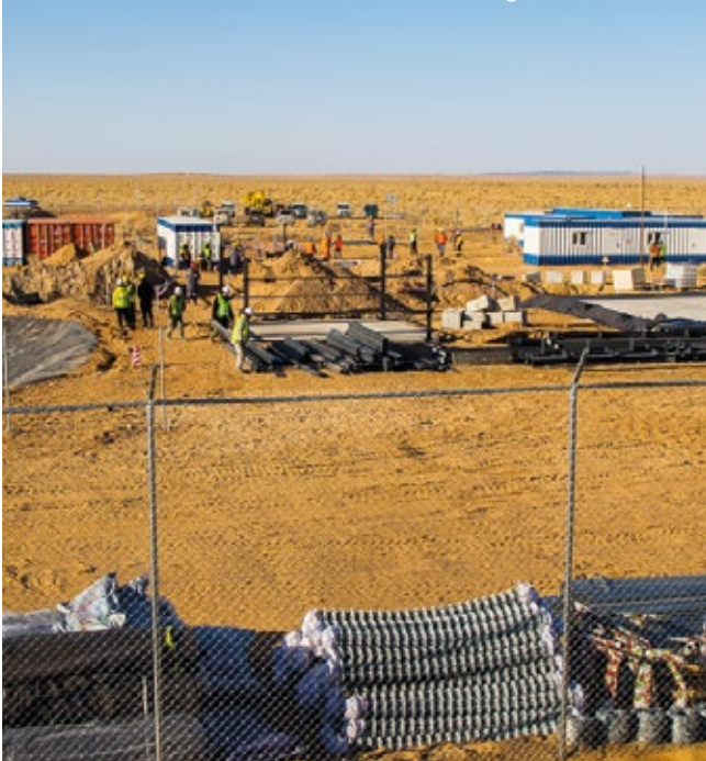
Zuuvch Ovoo ISR Pilot's construction works, Mongolia.
