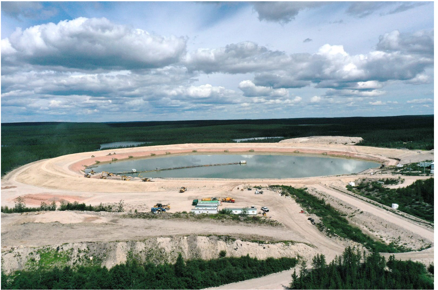
Figure 2.4 The JEB TMF at the McClean Lake Operation, Looking North
