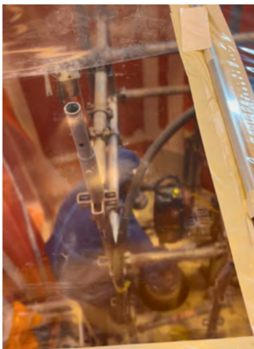
Photo 4 : carottage dalle silo HAO
