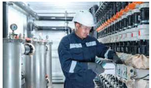
Well-house – internal view
