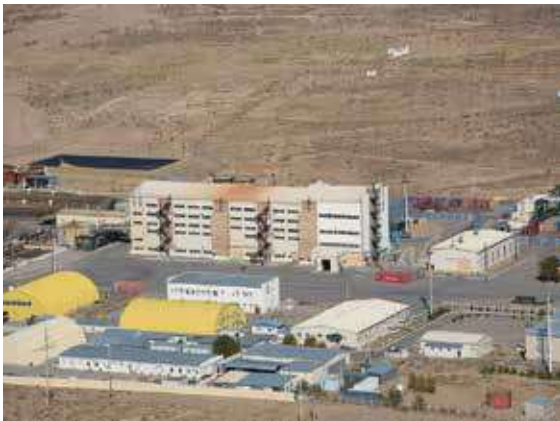
Tortkuduk processing plant, KATCO site, Kazakhstan
