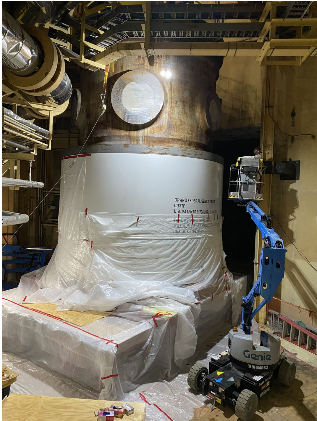
Image: The first piece of Crystal River 3's reactor vessel was lowered into a custom-built package for eventual shipment to disposal.
