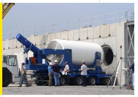
Getting ready to load canister from transfer cask into HSM.
