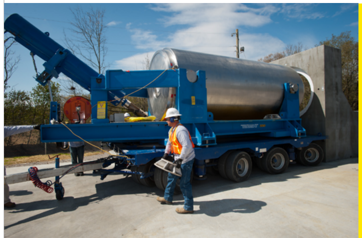
Inserting DSC into HSM Mockup
