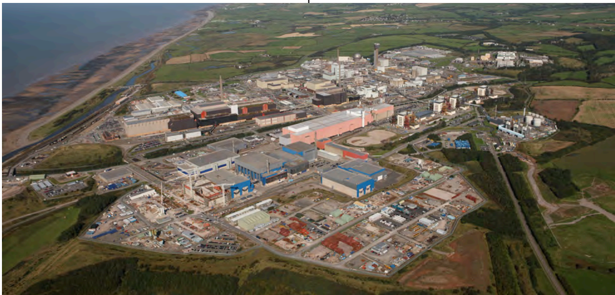
Aerial view of the Sellafield site where LEOPARD was integral in the RAHF D&D project. BNFL, England. ©2009 SELLAFIELD LTD
