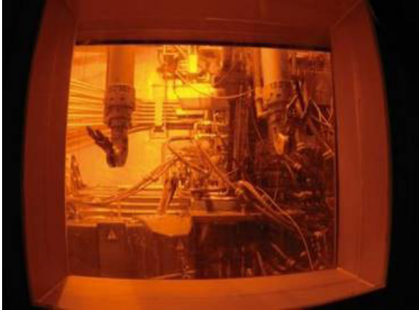
CCIM hot cell at La Hague R7 vitrification facility
