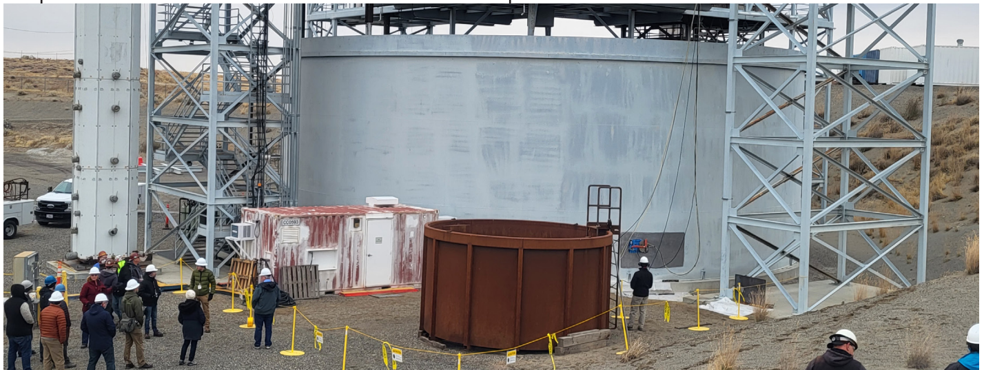
The Orano team performing a cold spray demonstration at Hanford's Cold Test Facility
