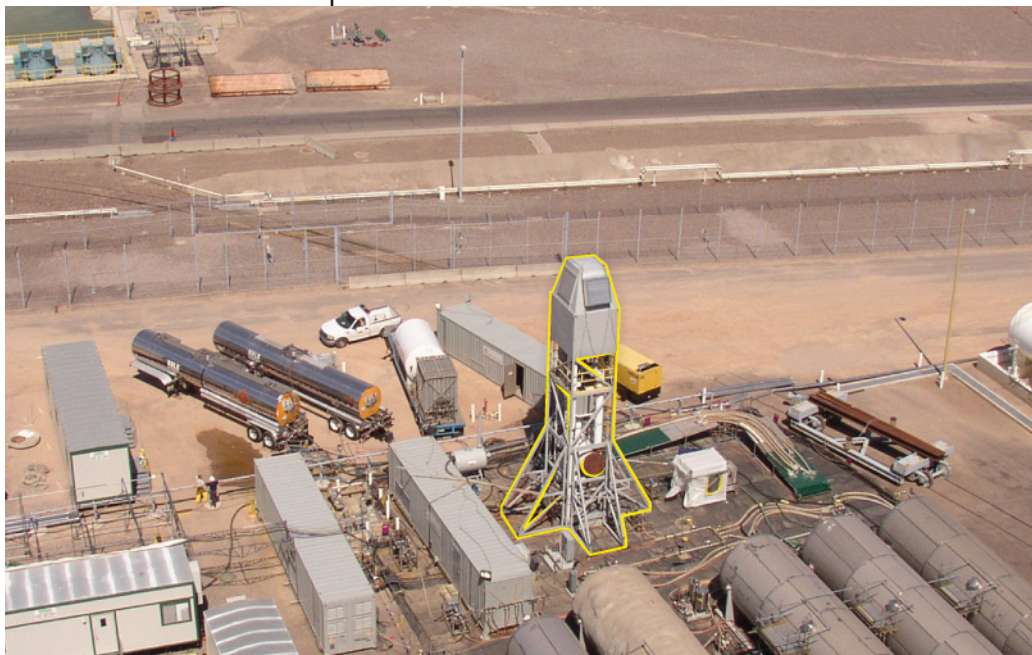
Mobile evaporator at Palo Verde Generating Station, Tonopah, Arizona
