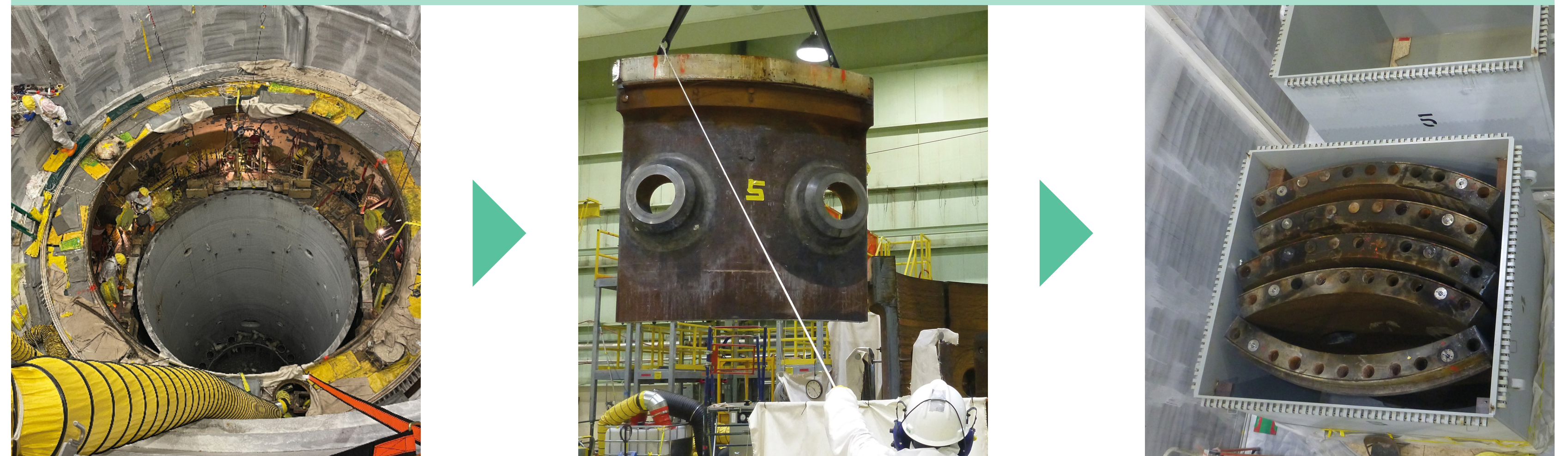
Reactor vessel segmented with mechanical and thermal cutting
