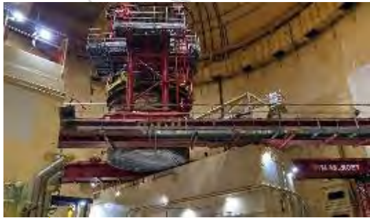
Reactor vessel segment handling in containment
